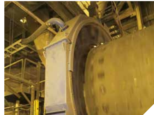
Protecting the gear with a pressurized guard
