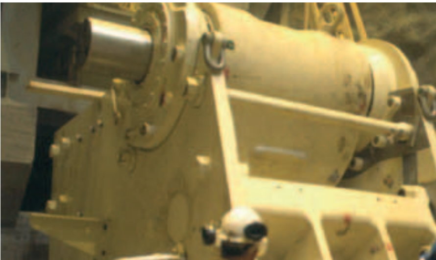
A Nordberg C200 jaw crusher being assembled at an underground mine. The crusher was transported in pieces and assembled underground.
