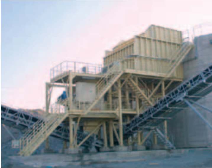
A C125 during the installation phase at a new primary crushing plant.
