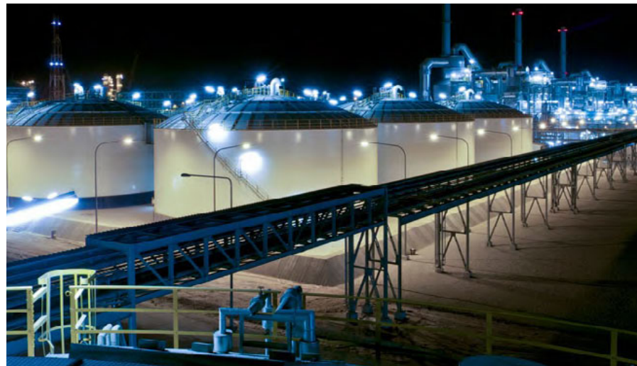
The world's largest sulfuric acid plant complex was built for Ma'aden in Saudi Arabia using Outotec technology. Ma'aden will also use Outotec-Hatch technology in its aluminum plant project.
