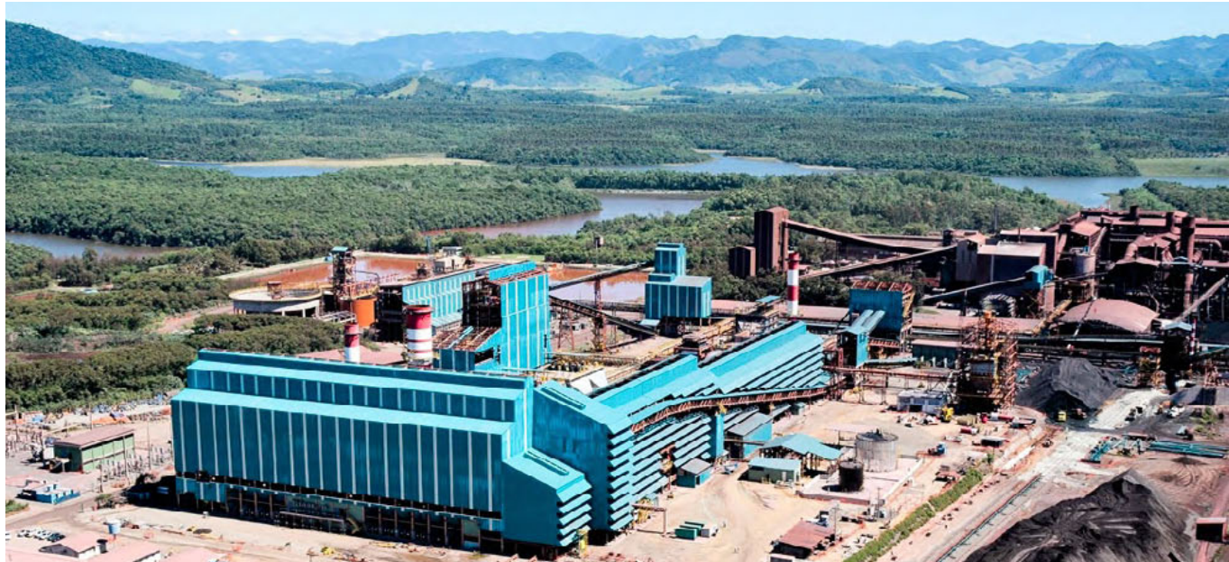
About two-thirds of the global pellet production derives from Outotec's leading technology with guaranteed high quality and low operational costs. Samarco in Brazil is the world's largest pelletizing plant with annual capacity of 7.25 million tonnes.
