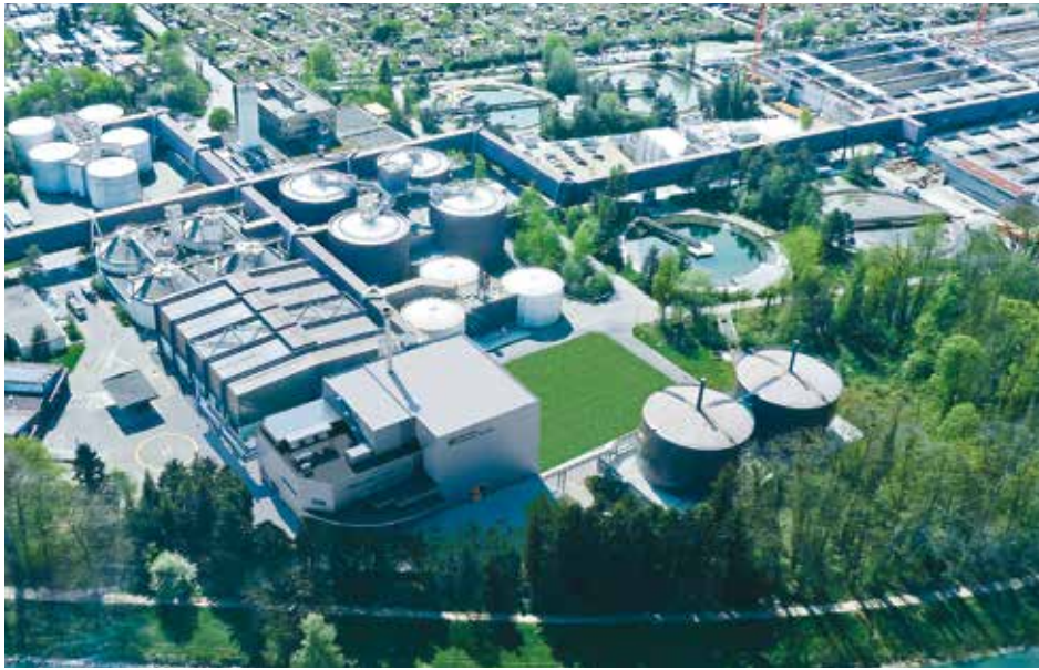
The Sewage Sludge Incineration Plant in Switzerland designed by Outotec operates as a self-sustained process, without external fuel. It can produce a surplus of electrical power or heat, and complies with all emission standards.
