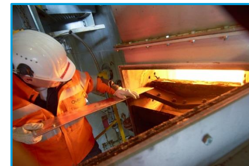
Waste to energy plants
