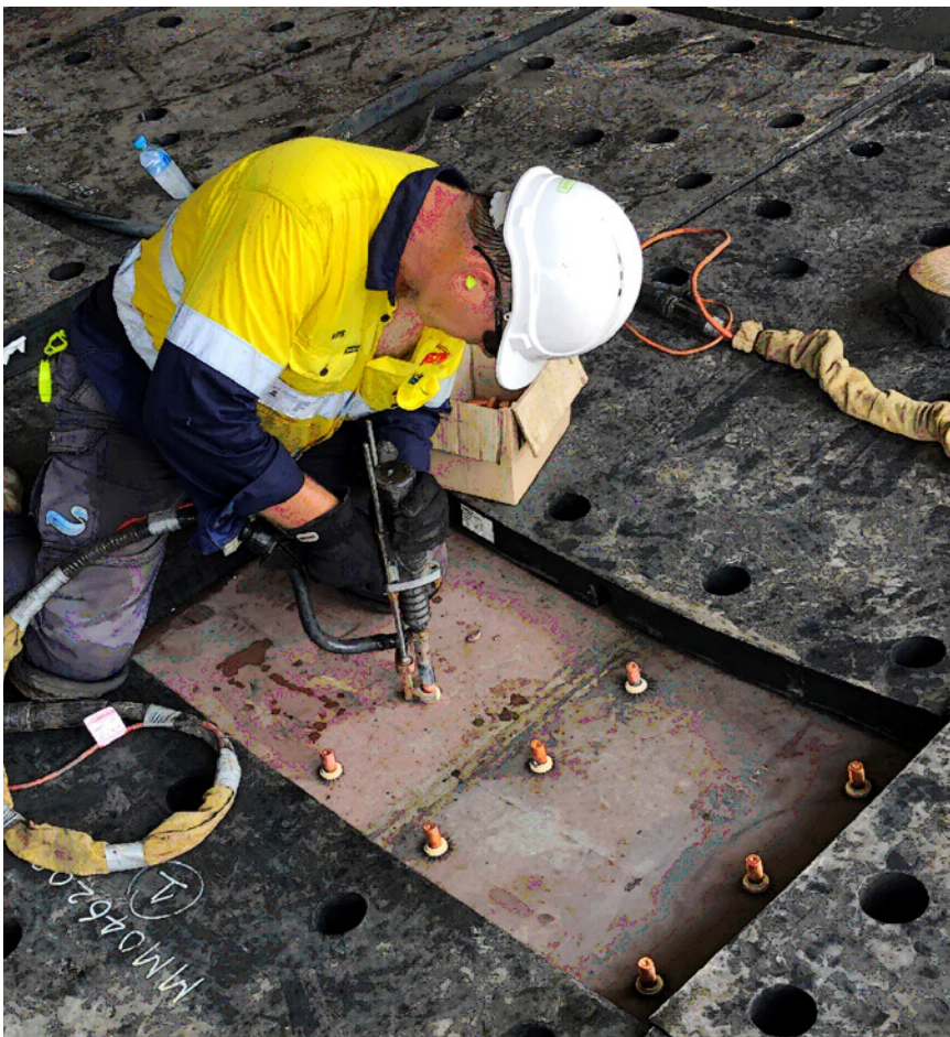
Typical fixing parts including stud bolts, washer, nut and rubber plug
