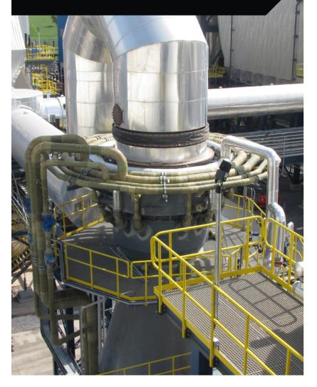
Metso OtoVent provides efficient and reliable quenching for hot corrosive process gases in wet gas cleaning plants. The system improves the reliability and performance of downstream equipment operation and prolongs its lifetime. Metso OtoVent is a flexible solution that can be customized according to the needs of your application.
