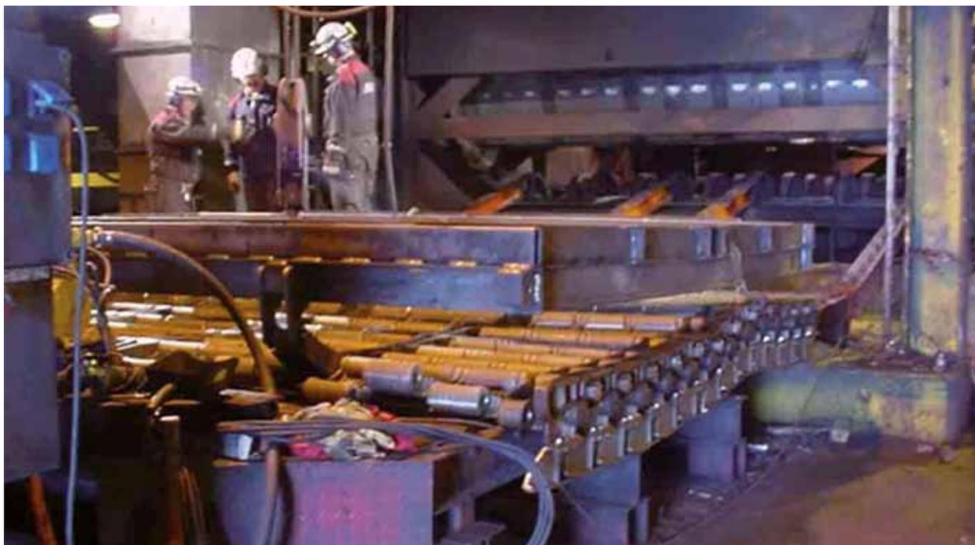
Installation of conveyor chain "Blanket" into travelling grate
